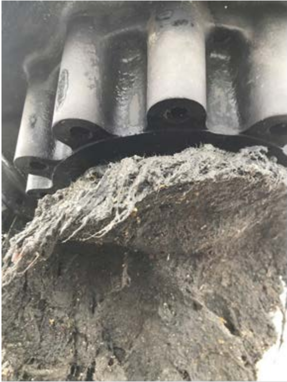
Debris clogging pipe
