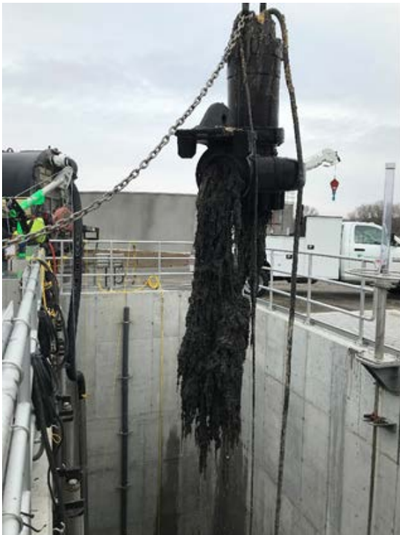
Debris clogging pipe
